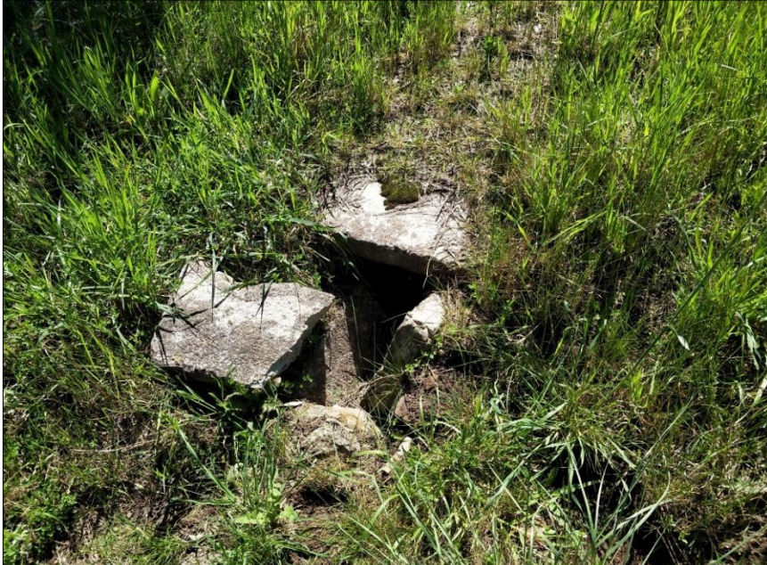
15: DILAPIDATED DRAINAGE INLET IN HISTORICAL COTTAGE AREA
