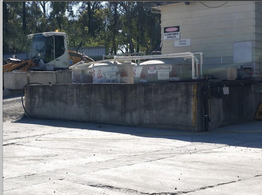
24: BUNDED 4,500 L CAPACITY ABOVEGROUND STORAGE TANK, FACING NORTH EAST. POTENTIAL LEAKAGES ARE EVIDENT ON THE RIGHT WALL.
