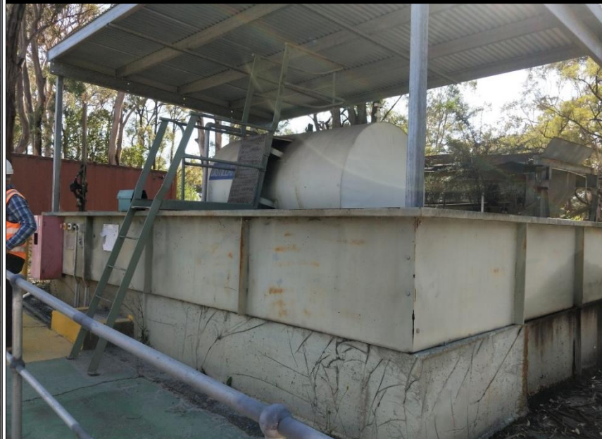
24: BUNDED 4,500 L CAPACITY ABOVEGROUND STORAGE TANK, FACING NORTH EAST. POTENTIAL LEAKAGES ARE EVIDENT ON THE RIGHT WALL.
